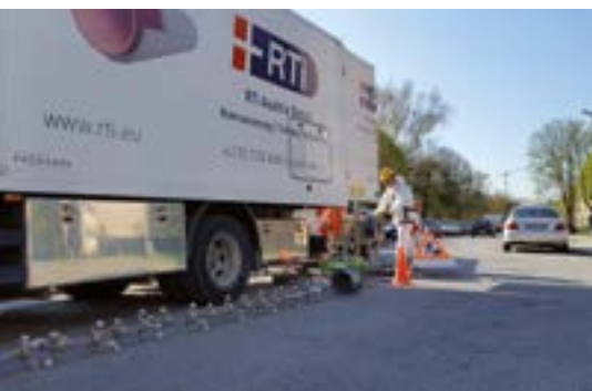
GRP liner installation
