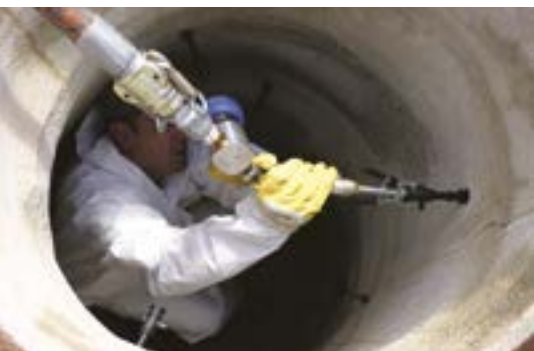
Cement paste injection in low pressure process
