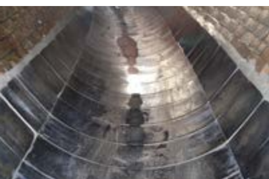
Lining with pipe segments
