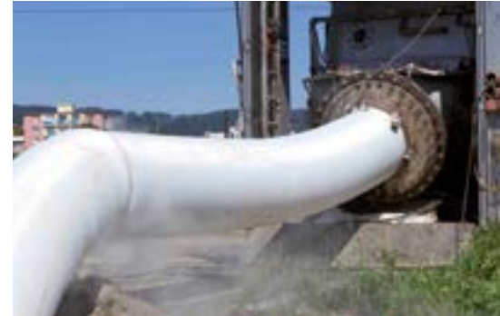
CIPP liner installation
