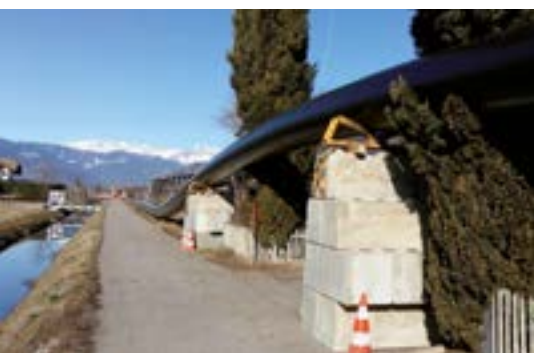
Lining with continuous pipe
