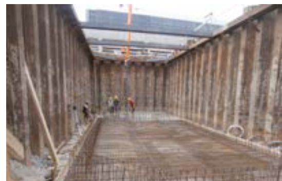
Excavation of a fat separator
