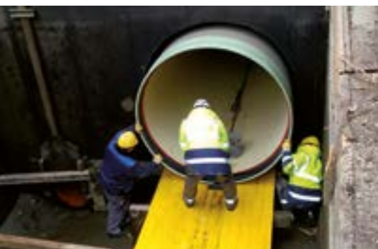
Lining with discrete pipes
