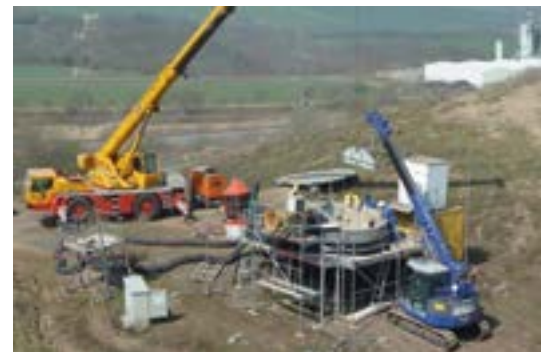
Inspection at landfill
