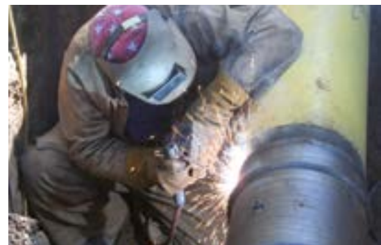
Welding work on gas lines
