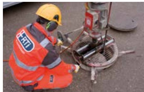
Manhole frame rehabilitation
