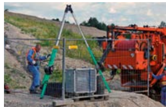
Elimination of encrustation at landfill
