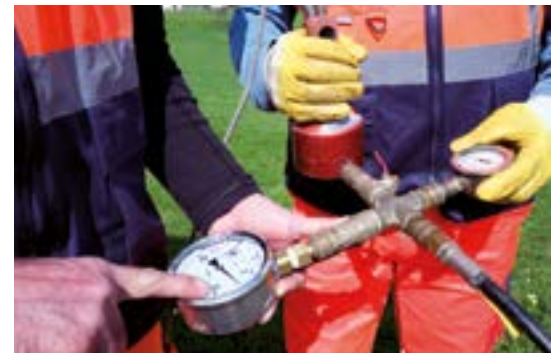
Pressure testing of a gravity pipeline
