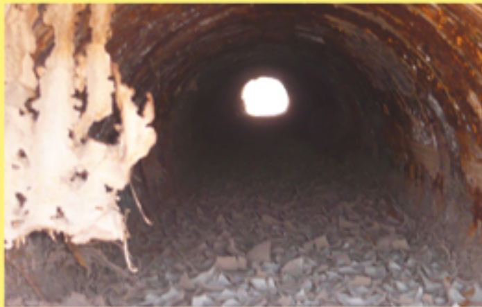
Corrosion-damaged oval-shaped CMP culverts are one of the many challenging problems that can be repaired with StifPipe™.
