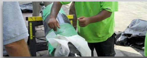
The PipeMedic™ assembly is held in coiled position using strings or rubber bands
