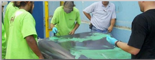
The outer surface of PipeMedic™ is also coated with epoxy for bonding to the interior surface of the pipe
