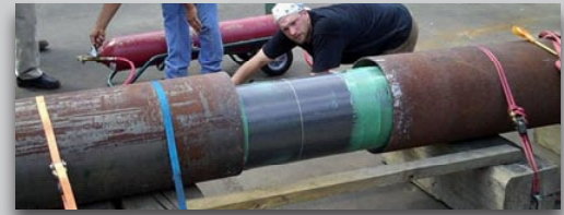
The packer is inflated, allowing the PipeMedic™ to unwind ...
