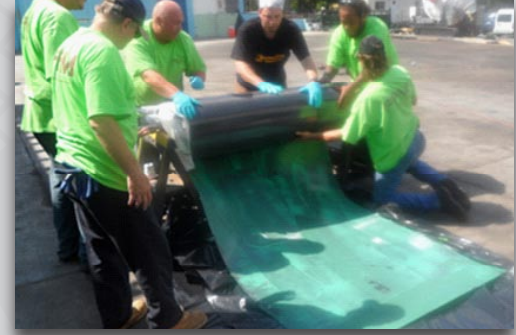
PipeMedic™ laminate is rolled up around the packer into a coil with a diameter of approximately 12 inches (300 mm)
