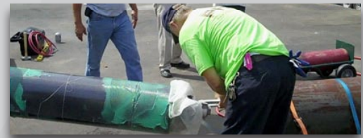
The PipeMedic™ and packer assembly is inserted into pipe ...
