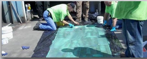
PipeMedic™ PC26.16 laminate is cut to length and QuakeBond™ J201TC epoxy is applied to one face.
