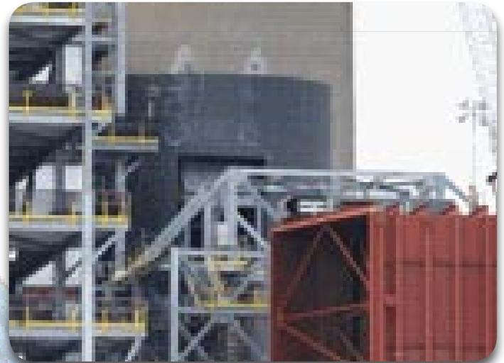
Concrete has been removed in anticipation of placing duct work.
