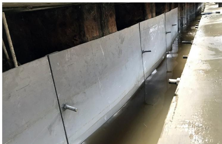
The Sheet Pile Repair (SPIRe®) system is an innovative new system of **repairing and restoring corroded steel sheet piles**, both above and below water, using FRP composites\*
