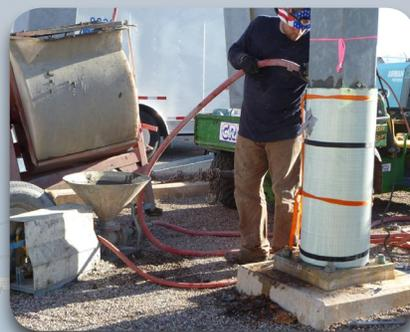
Fill the annular space with grout & vibrate
