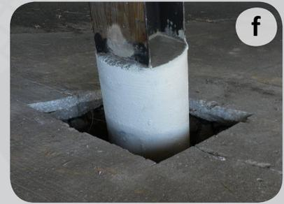
a. Corrosion-damage   b. Apply epoxy to PileMedic™   c. Wrap PileMedic™ around column or pile to create a cylindrical shell
