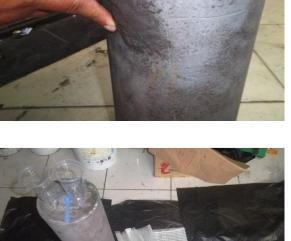
Wrap the saturated fabric around the pipe to cover the area where the hole. Note that the fabric overlaps around 6 inches (150 mm).
