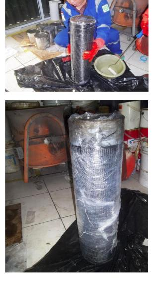
12. The ends of the pipe were capped, sealed and filled water. An initial pressure test was performed to make sure there were no leaks in the system.
