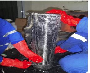
10. If necessary, apply a top coat of QuakeBond<sup>™</sup> J333SR to the carbon fabric to make sure the fabric is fully saturated.
