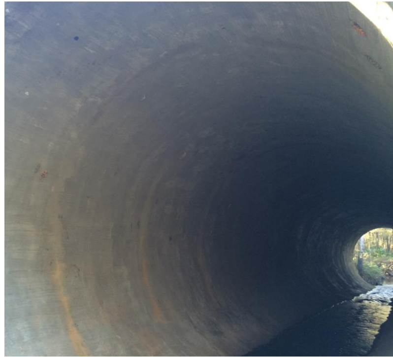
Figure 3: Six-year visual inspection - No visible wear, voids, or fractures
