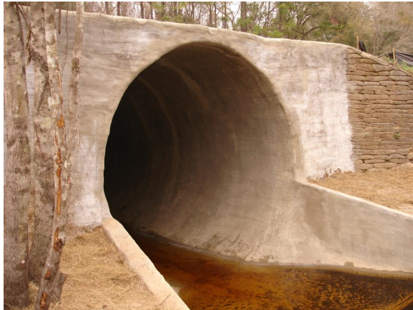
Figure 2: Fully structural, smooth, watertight rehabilitated culvert
