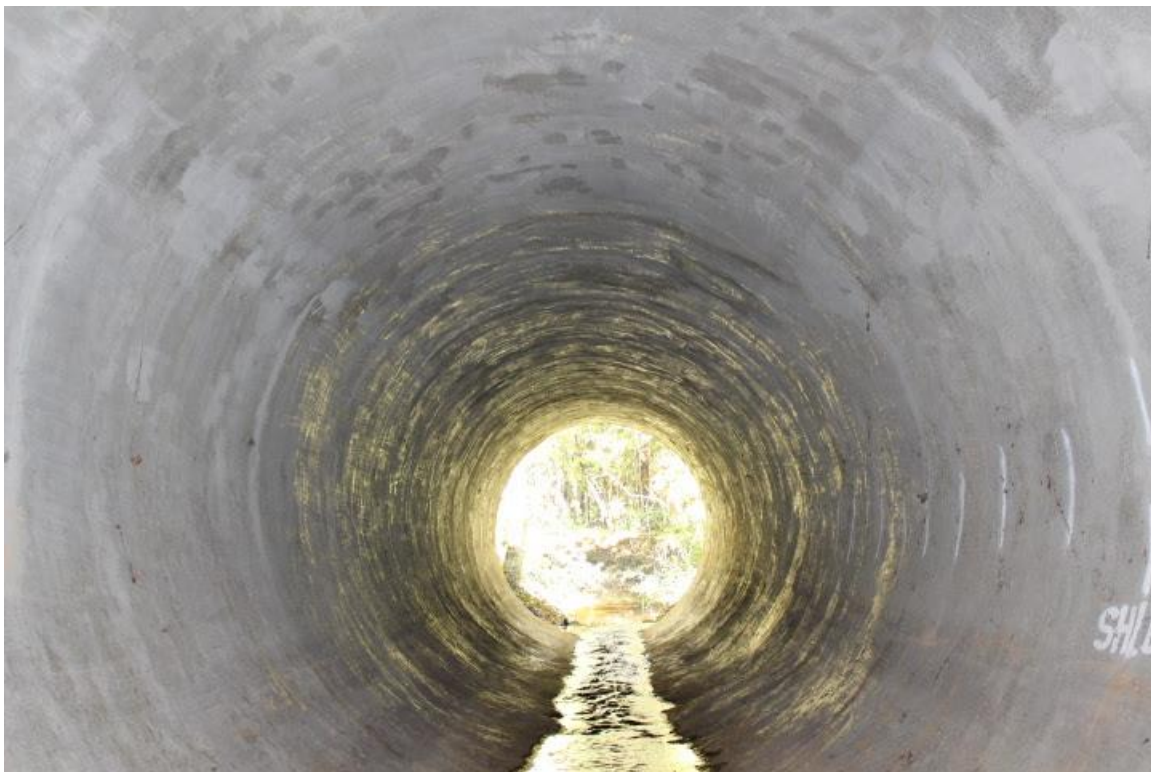
Figure 14: November 2016 - Photo of structurally sound rehabilitated pipe, taken during strain gauge testing.
